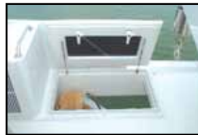
Ladderwell hatch, Proud coaming, Open, Exterior
