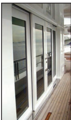
Bi-parting, Sidelights, Installed
