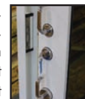
Two sets of handles, Top for latching, Bottom to cam door in and out against gasket
