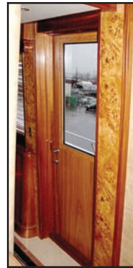
Interior view, Faux painted woodgrain
