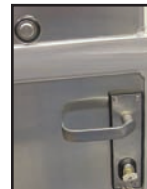
Blind dog, TrioVing® lockset with escutcheon plate, Exterior
