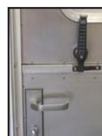
Interior view of blind dog, TrioVing® lockset, Adjustable
